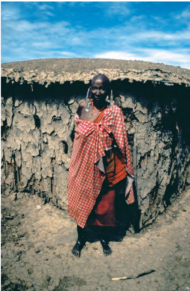
The Masai of Kenya have been using composite materials—mud, dung, and straw—to make homes for thousands of years.
