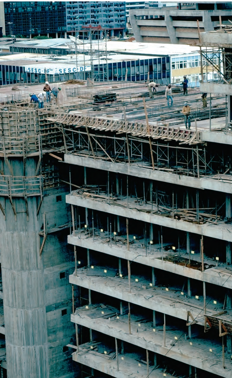
This skyscraper was built using a wide variety of mixtures, including concrete, steel, and glass.
