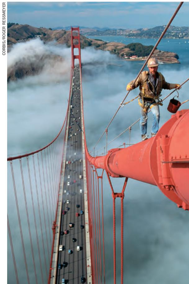
*Paint is applied to combat the rust problem. Paint prevents the iron in the steel from coming into contact with water and oxygen, the other reactants in the rusting equation.*
