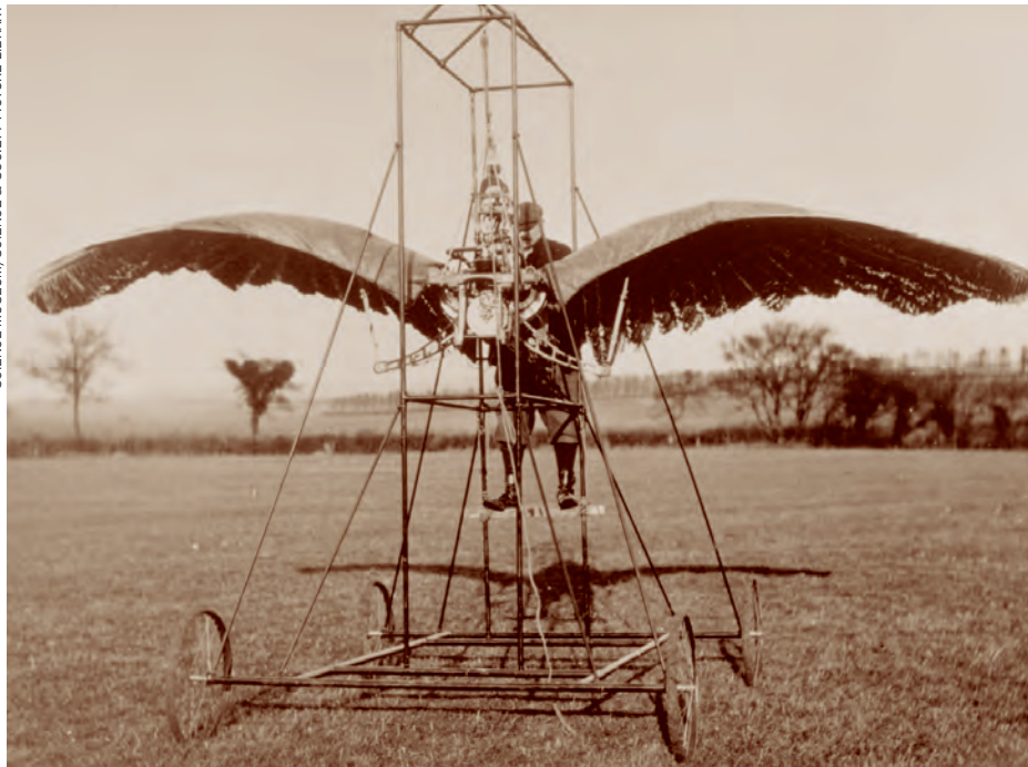
Many early attempts at human-powered flight, like that made in this ornithopter, failed because of poor design and the lack of strong, low-density materials.
