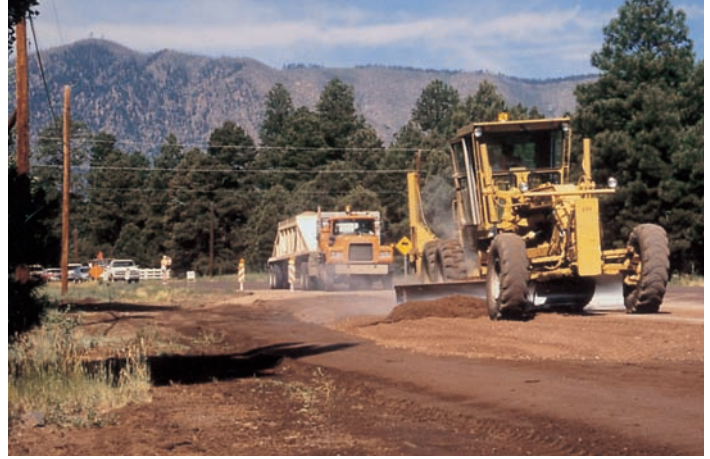
Roads and freeways are paid for with local, state, and federal tax dollars.
